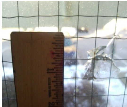
(Caulked bullet hole in chambers)
